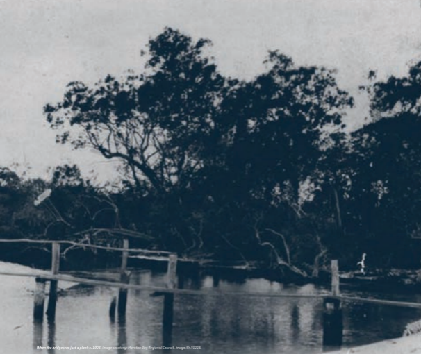
When the bridge was just a plank c. 1925. Image courtesy: Moreton Bay Regional Council, image ID: 71228.
